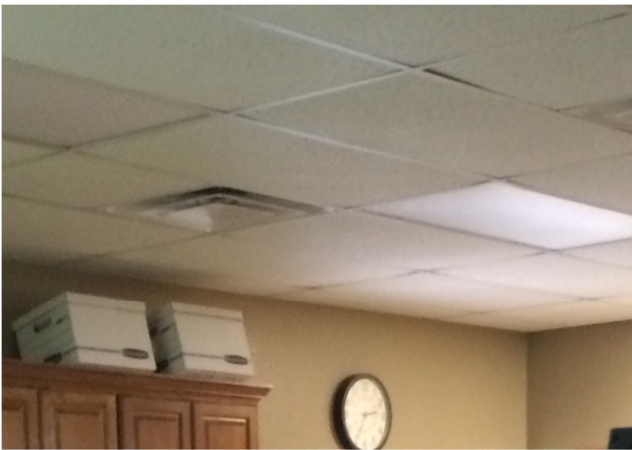
Figure 1. Photograph of lighting in Control Room “A”.
