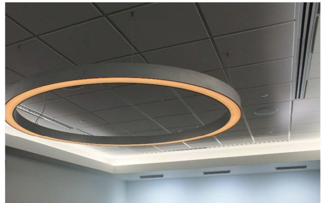
Figure 2. Photograph of lighting in Control Room “B”.
