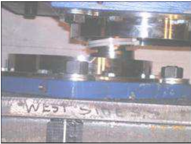
Fig. 1.2. Friction pendulum bearing with two sliding surfaces [3]
