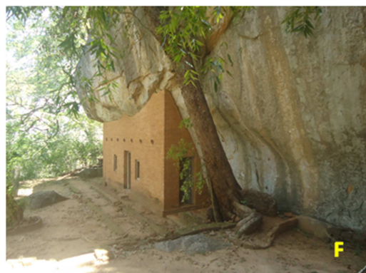
Boulder rock-shelters at Pidurangala (E & F) area. These shelters have valued as ancient monasteries and palaeolithic sites. Such valued many rock-shelters have been destroyed by newly constructed structures.
