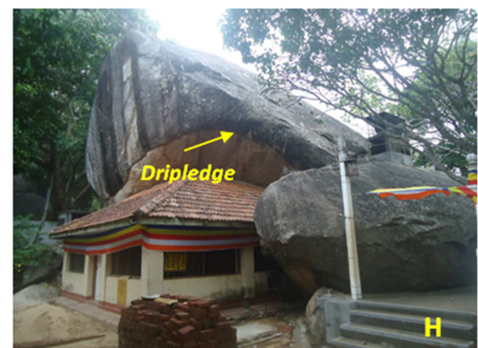
Boulder rock-shelters at Pidurangala (G) and Enderagala (H) areas. These shelters have valued as ancient monasteries and Palaeolithic sites and. Such valued rock-shelters have been damaged by newly constructed structures. These structures act as major barriers for deep excavations.
