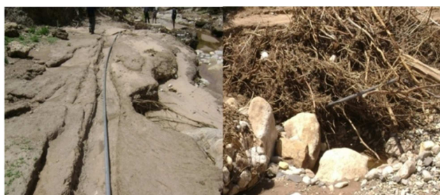
Fig. 3.11. Flood damage on potable water pipe lines.
