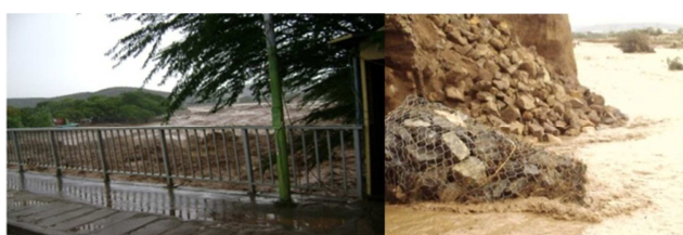
Fig. 3.12. Water level around Kezira main Bridge & Damages on gabion.
