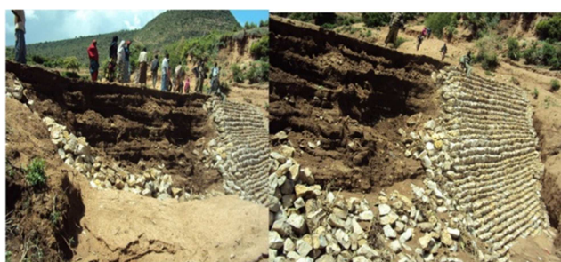
Fig. 3.13. Damages on Sediment Storage Dams (SSDs).
