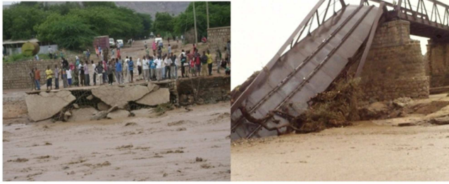
Fig. 3.14. Flood Damage on Hafkat ford and Damage on Railway Bridge.
