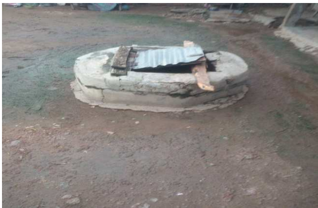
Figure 5. Improperly Covered well in the area.
