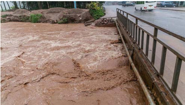
Figure 1. Nyabugogo bridge after a heavy rain on January 26, 2020, Source: NewTimes.
