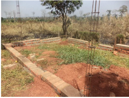
(a) Foundation of a house under construction using clay bricks.
