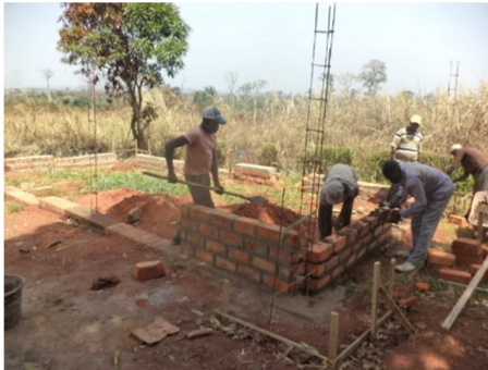
(b) Wall building of a house using clay bricks.
