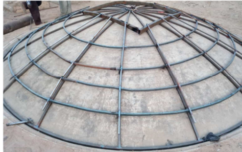
Figure 3. Constructed frame and the mold.
