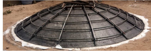
Figure 5. The steel frame and mold.
