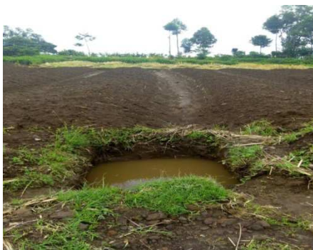
Figure 3. Traditional dam or water retention ditch.
